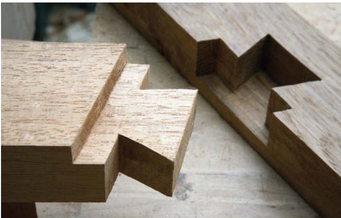
The underside of the dovetail is sawn away to one-third of its depth
