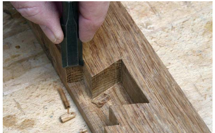
Socket is chopped and pared out with chisels to two thirds of the depth of the post
