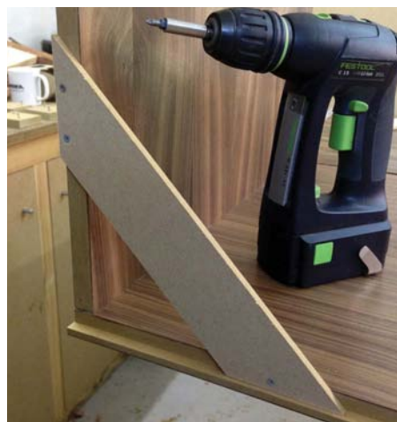
Fix temporary corner bracing to support the carcass
