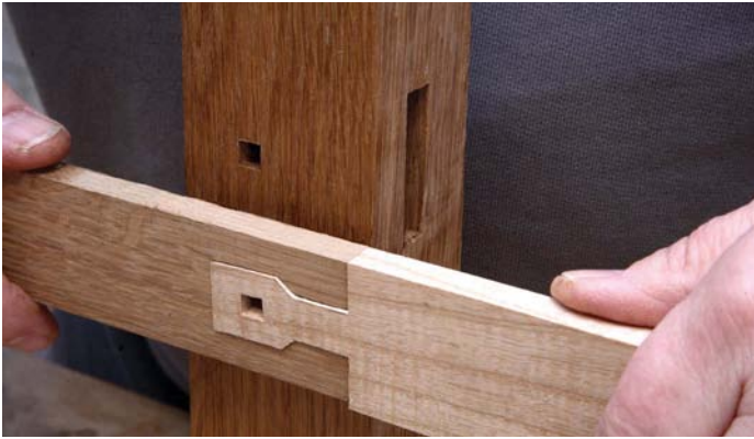
Gooseneck pin and socket are trial-fitted and the corner post – behind – has a mortise socket chopped through it ready to receive the gooseneck parts
