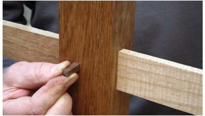
Assembled gooseneck jointed rails are slid through the mortise socket and the pin is inserted through both sockets in post and the gooseneck, completing the Komisen-uchi joint
